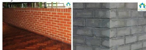
Fig.3: CLC blocks wall
