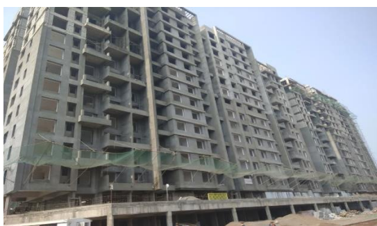
Fig 5: Plastering at site
