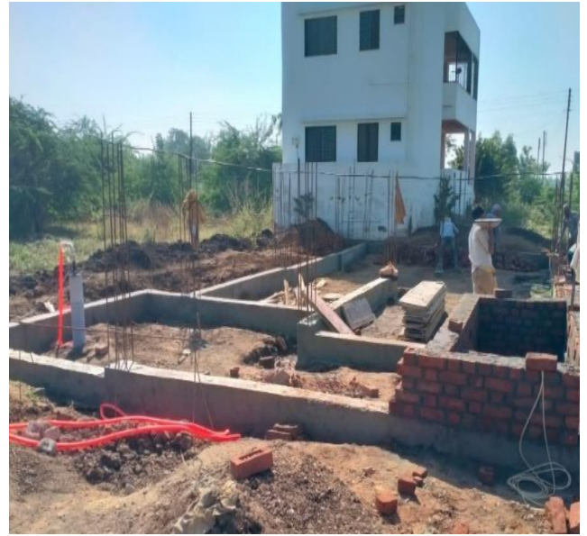
Fig.6: Ground Beam
