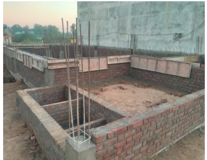
Fig.7: Brick work and casting of plinth beam
