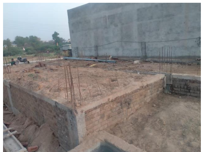
Fig.8: Backfilling
